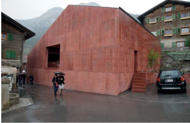
OBR. 3 Valerio Olgiati, Atelier Bardill, Scharans, Švýcarsko, 2007 – foto: FŠ FIGG. 3 Valerio Olgiati, Bardill Atelier, Scharans, Switzerland, 2007; Photo: FŠ
