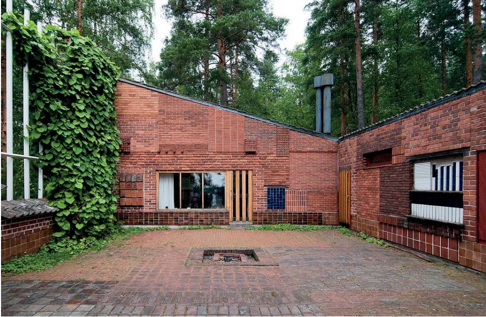
OBR. 2 Alvar Aalto, Experimental House, Muuratsalo, Finsko, 1954 – foto: Ivan Himanen FIG. 2 Alvar Aalto, Experimental House, Muuratsalo, Finland, 1954; Photo: Ivan Himanen
