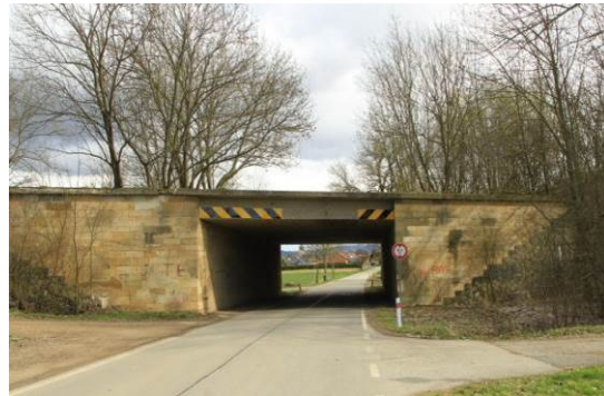
Fig. 3: Bridge over road W of Jevíčko
