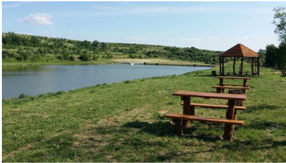
Fig. 1: Water reservoir Nenkovice with a resting point
